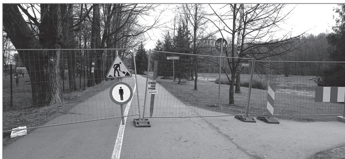
Na bulwarach remont.
